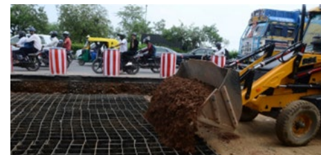
Use of Geocells prepared from waste plastic in road construction
