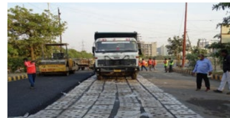
Use of waste plastic modules in road construction
