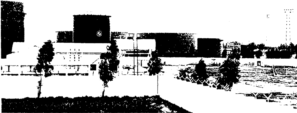
This new BPC installation at Bijwasan is representative of the expansion of the Corporation's distribution network
