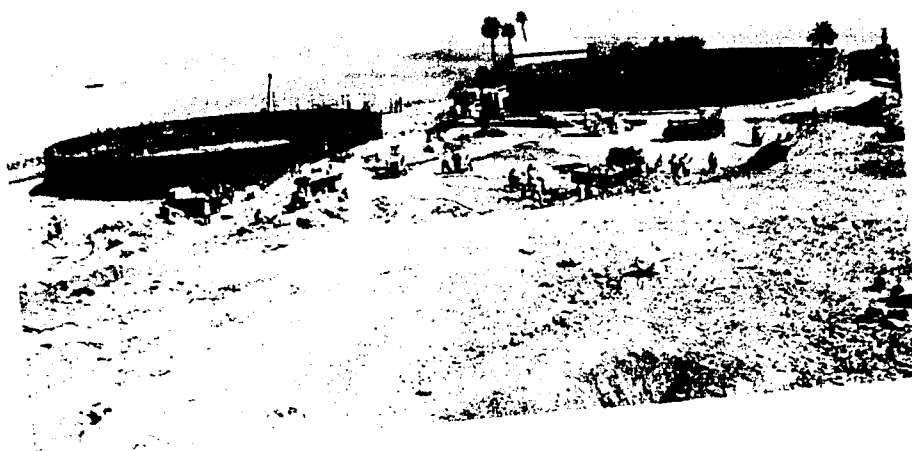
Six tanks with a total capacity of 1,62,000 Kls will constitute the new tankage on Butcher Island. Here we see two of these tanks taking shape.
